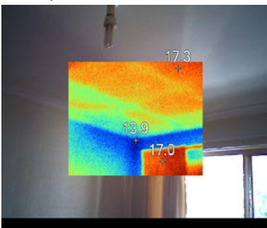
Insulated ceiling and uninsulated wall
