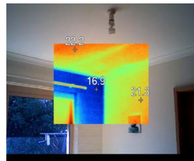
Internal and external walls 5 October 2012, 10:45:31am
