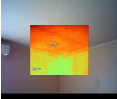
Main bedroom, south corner, ceiling 5 March 2012, 10:28:37 am
