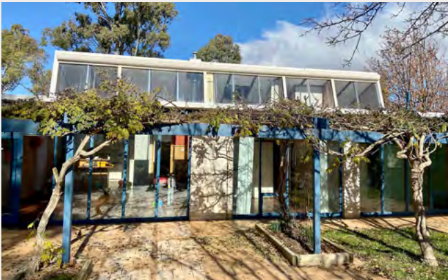
↑ Kalma House in 2021, designed by Derek for two CSIRO scientists and built in 1977. The Light House team were delighted to be contacted by the new owners who were seeking advice on how to renovate the home while honouring its original excellent solar passive design. Image: Jenny Edwards
